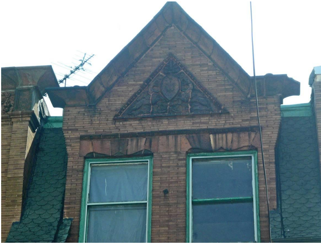
Figure 7: Detail of 3 rd story wall dormer.
