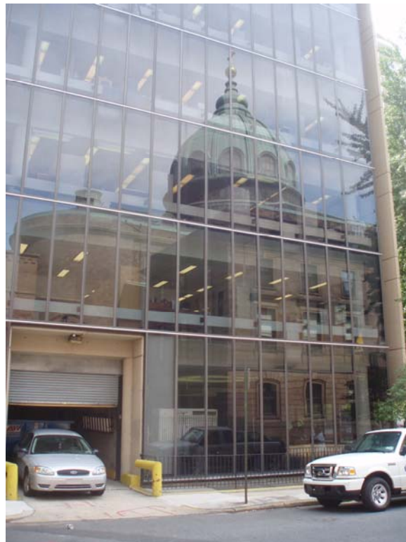
Figure 10: North elevation detail (September 2010)
