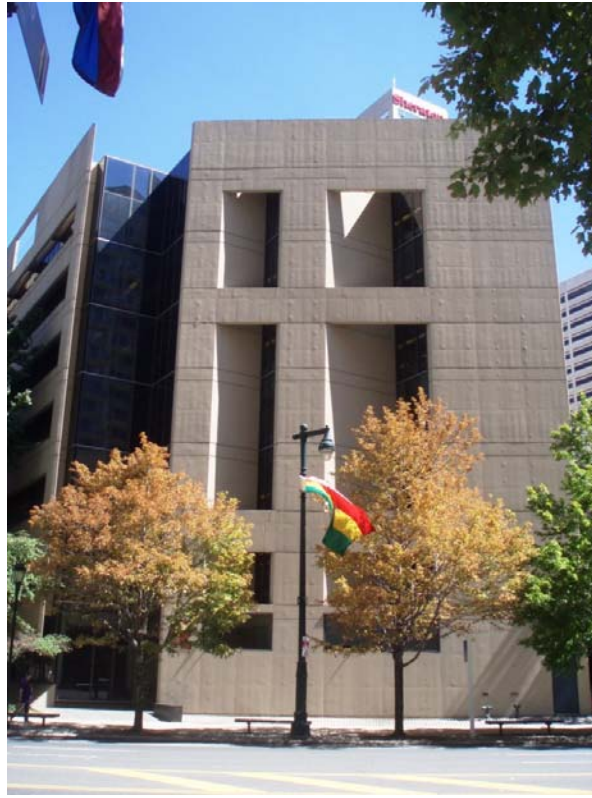
Figure 3: South elevation (September 2010)
