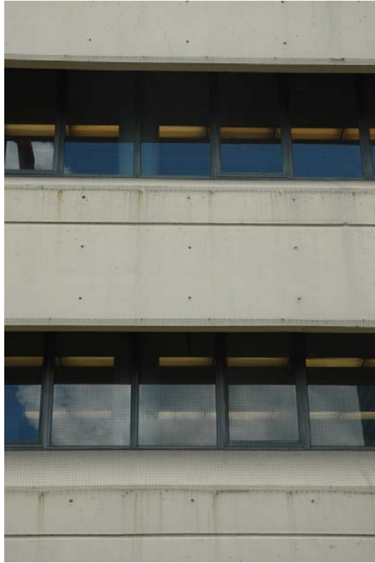
Figure 7: West elevation detail (September 2010)
