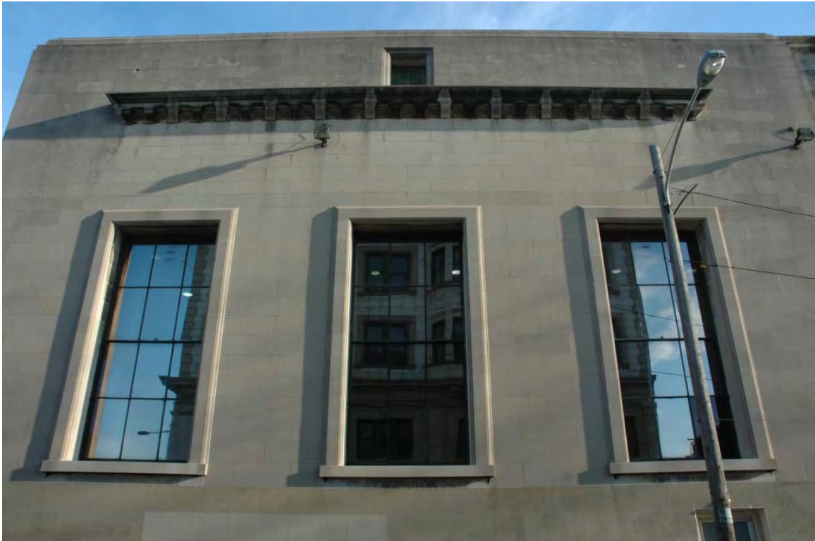
Figure 9: South elevation window and cornice detail.
