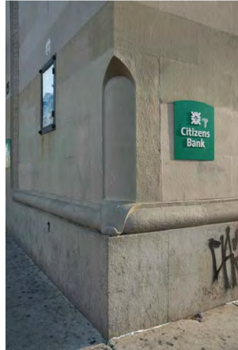
Figures 6, 7: Detail of west elevation painted granite base, door surround moldings, and contemporary bank signage (L); Detail of chamfered southwest corner (R).
