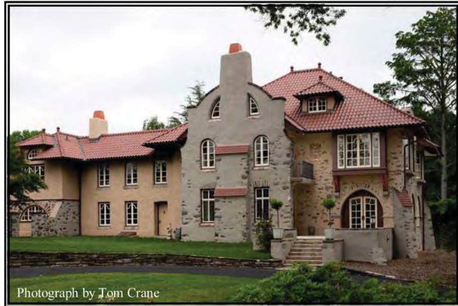
Schoen Estate Renovation circa 1904 William L. Price Architect
