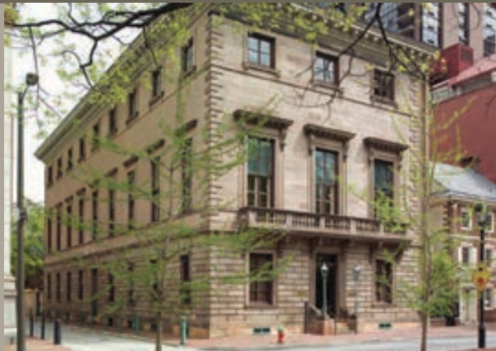
Photography © Tom Crane, 2006
