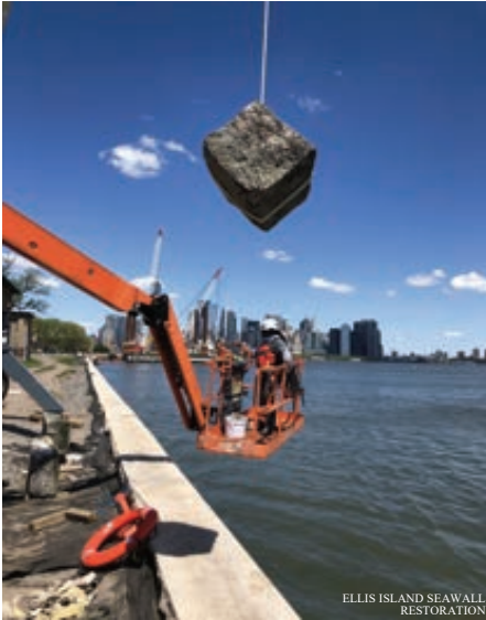
ELLIS ISLAND SEAWALL RESTORATION
