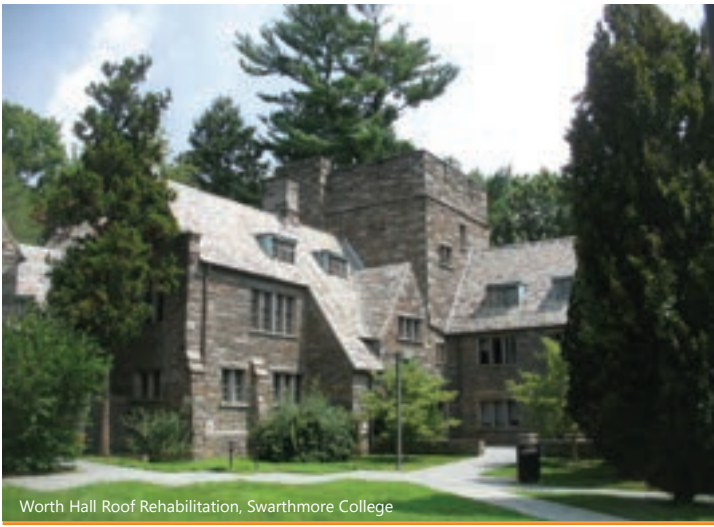
Worth Hall Roof Rehabilitation, Swarthmore College
